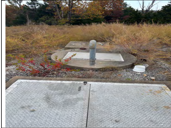
City of Lake Ozark wastewater infrastructure. No active operation or connection
