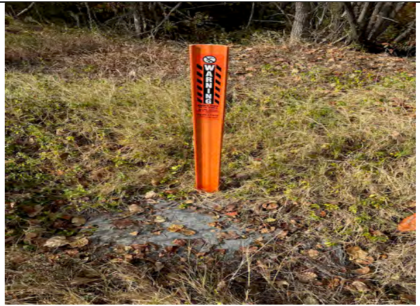
Marked fiber cable in NW corner
